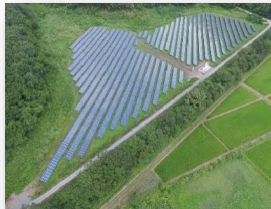
View of the SW section of the plant
