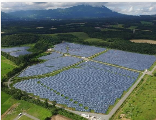
General aerial view of full plant
