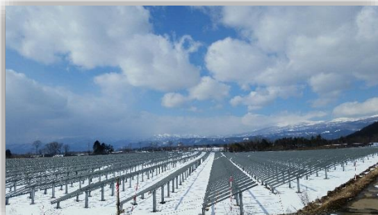
View of fix-tilt structures
