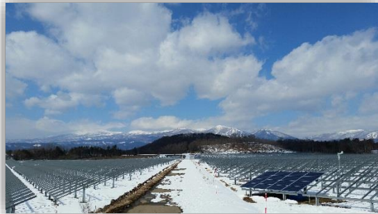
General view of the plant
