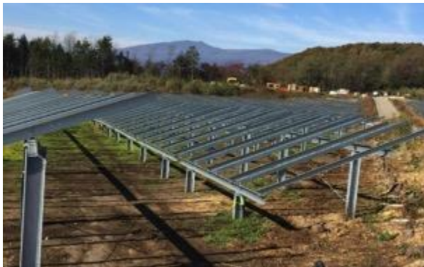
View of fix-tilt structures
