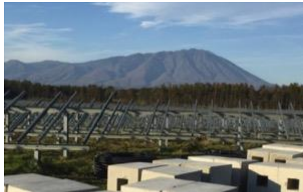
General view of plant
