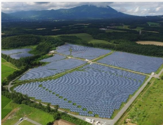
General aerial view of full plant
