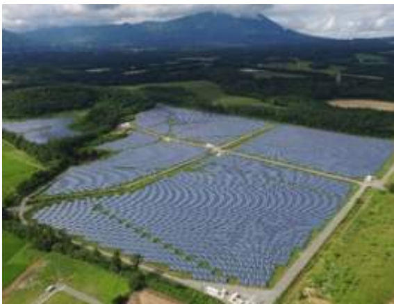
General aerial view of full plant
