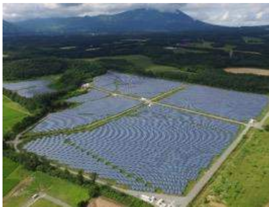
General aerial view of full plant
