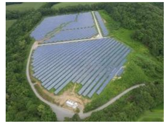
View of the NW section of the plant.
